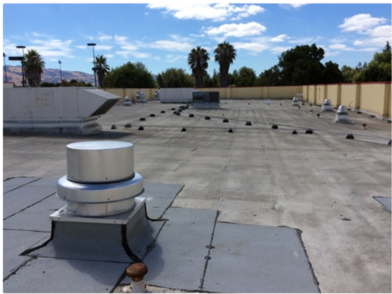
An overview photo from the roof level.
